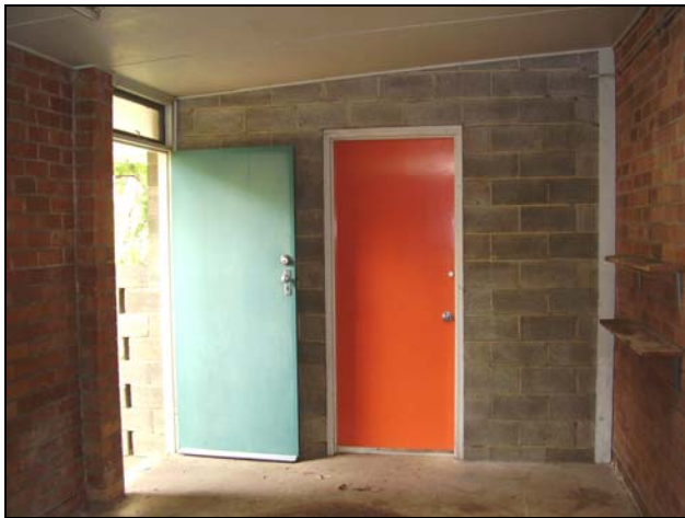
Figure 3.68 The garage has brick and concrete block walls with constructed on a suspended concrete slab. A workshop is located at the western end.
