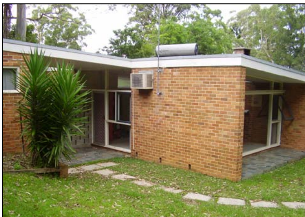
Figure 3.19 The rear of the living wing which features glazed walls with flush timber doors and paved terrace and porch areas.
