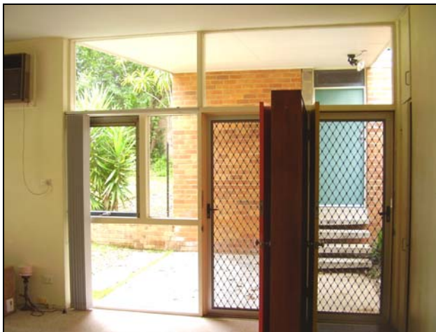
Figure 3.43 The bookshelf unit also forms part of a glazed wall which provides visual and physical connection to the entry and adjacent covered terrace.
