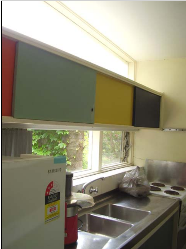
Figure 3.47 Cabinets and kitchen window. The cabinets correspond to the coloured solid panels facing the service courtyard.
