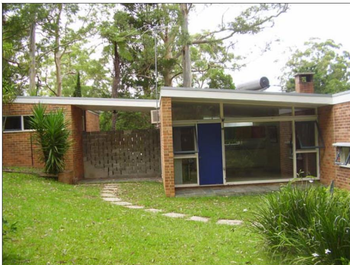
Image 4 – Photo rear facade (Source: PMA 2015)
