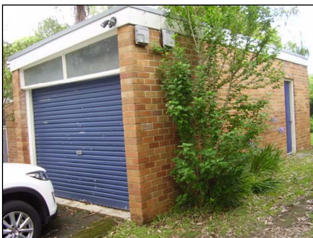
Figure 3.15 The house roof is continuous and extends over the garage wing which has simple flush doors on the northern and southern walls and a roller door with timber framed infill over facing the street.
