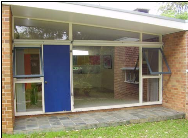
Figure 3.21 The glazed wall and door in the living room.
