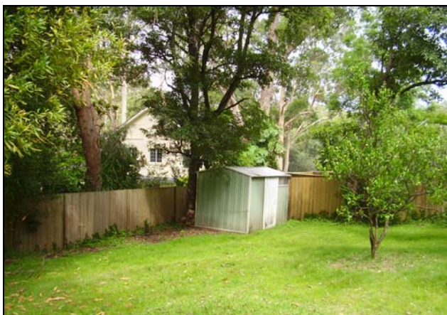
Figure 3.33 A simple, small steel shed is located in the south western corner of the site.
