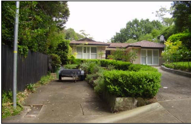
Figure 3.10 Further north No. 25 Finlay Road is a modified single storey dwelling with hipped roof clad in tiles.
