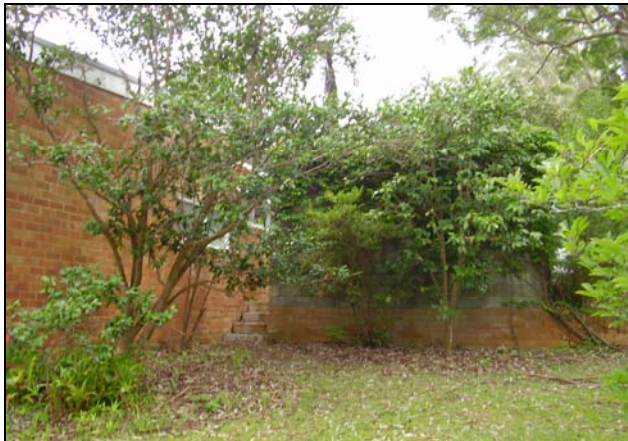
Figure 3.35 The front, service courtyard conceals part of the front façade of the building.
