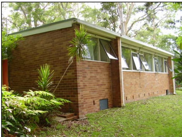
Figure 3.25 The southern facade of the building (and bedroom wing). Each bedroom and ensuite have fixed and hopper timber framed windows on solid brick base between the projecting end blade walls.
