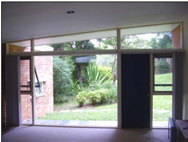
Figure 3.50 An original timber framed glazed wall with flush timber door provides visual and physical connection to the rear yard.
