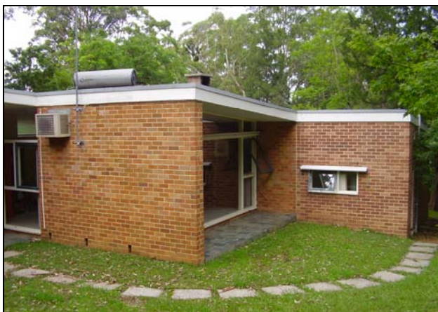
Figure 3.22 The rear of the house. A number of minor additions are visible including curved path (paving), air conditioning unit and solar heating panel also the ensuite addition at the western end of the bedroom wing (south western corner of the house).
