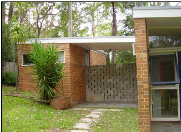
Figure 3.18 The rear of the garage wing and concrete block wall which extend between and connect the house and garage and also frames the building entry.
