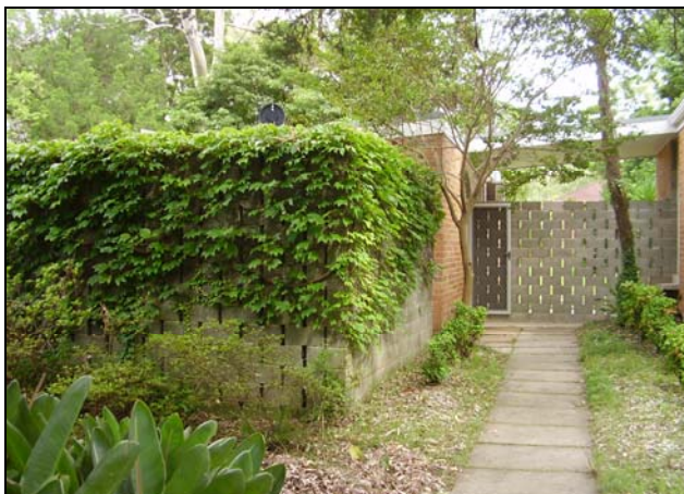
Figure 3.37 The service courtyard/ drying yard is also accessible from the pathway extending to the building entry.
