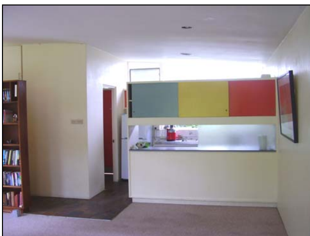
Figure 3.44 Original kitchen cabinets and “furniture” including servery with coloured and translucent sliding panels remain and allow both separation and connection between the kitchen and open plan dining and living area.
