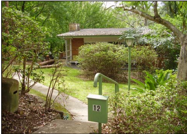
Figure 3.2 Diagonally opposite the site, No. 12 Finlay Road is a single storey Post-war brick dwelling with low pitched skillion roof clad in metal sheeting and stone chimney.
