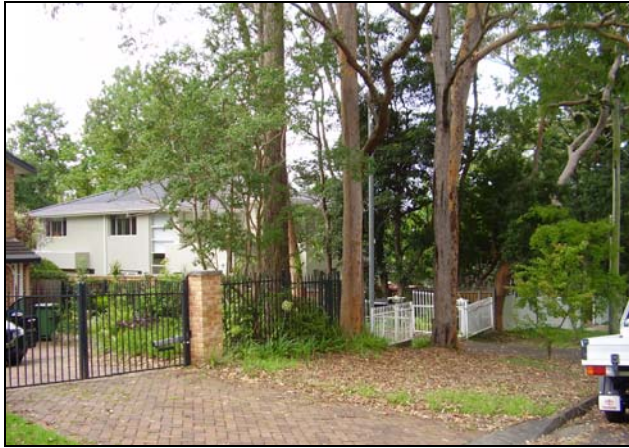
Figure 3.6 No. 24 Finlay Road is a rendered, late 20 th century two storey dwelling with hipped and gable roof clad in tiles. The buildings are all set back from the street frontage with gardens located between.
