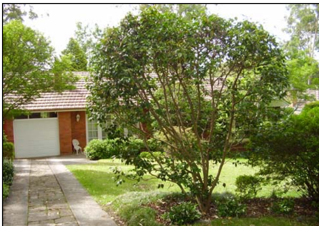
Figure 3.3 Located opposite the site, Nos. 14 and 16 Finlay Road are also single storey face brick Post-war detached dwellings with gable and hipped roofs clad in tiles.
