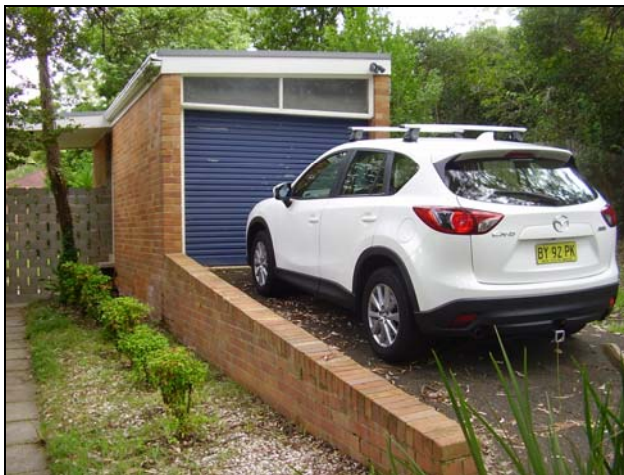
Figure 3.14 A driveway extends from the north eastern boundary to the garage wing which is elevated above the level of the house. A graded brick retaining wall also bounds the driveway.
