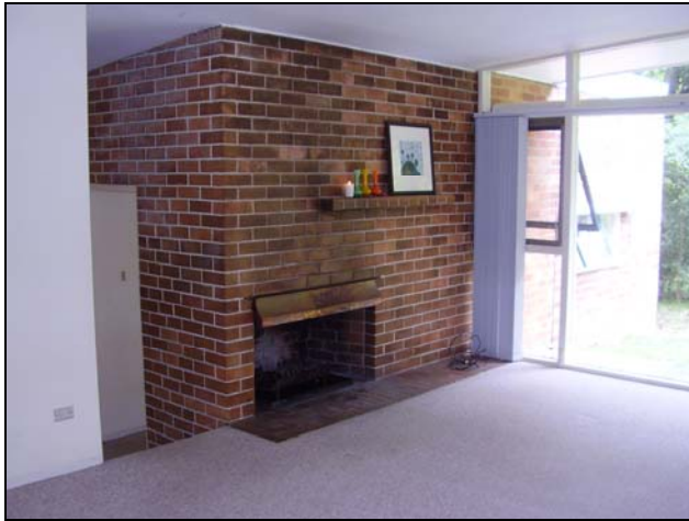
Figure 3.49 The living area retains the original face brick feature wall, fireplace and brick shelf. A small copper hood has been fixed over the fireplace.
