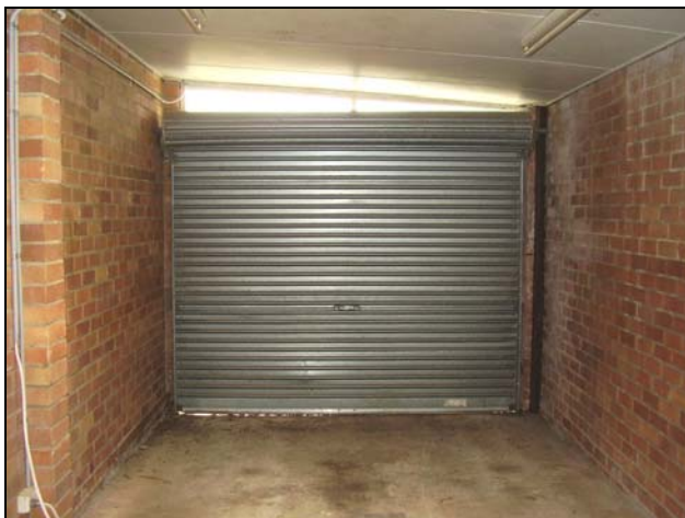
Figure 3.69 The garage also has a simple sheeted ceiling with surface mounted fluorescent lights and skylight and a roller door and toplight have been added to the eastern opening facing the street.
