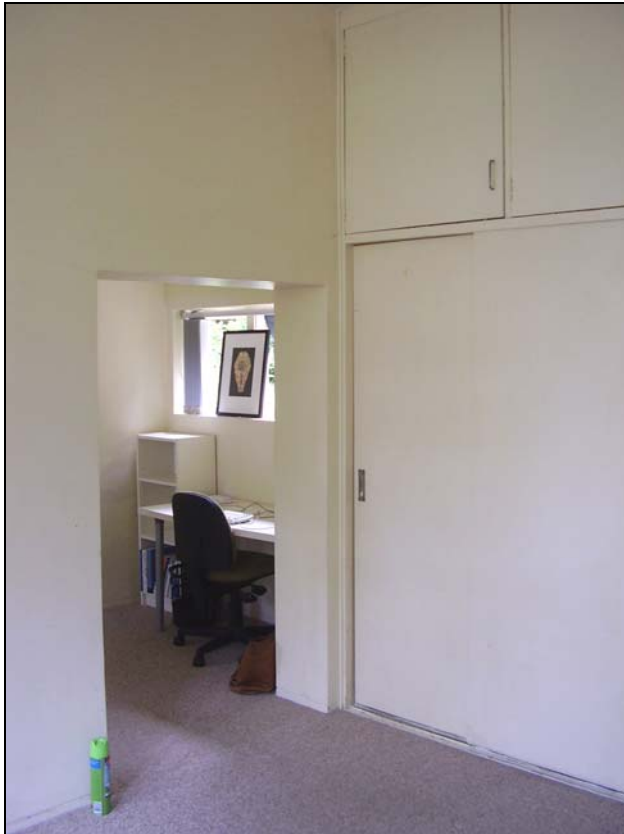
Figure 3.65 The built in cupboard and ensuite addition. A former window opening in the end wall (note the thickness) has been used to access the ensuite addition.
