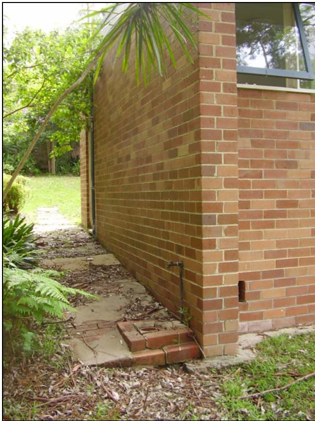
Figure 3.24 The end wall of the bedroom wing and ensuite addition. The addition, also designed by Harry Seidler & Associates is constructed of closely matching brick with similar details as the original house.
