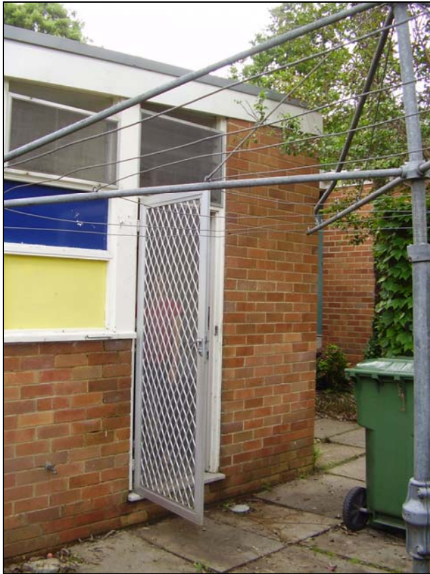
Figure 3.40 The laundry door. A flyscreen has been added to the door.
